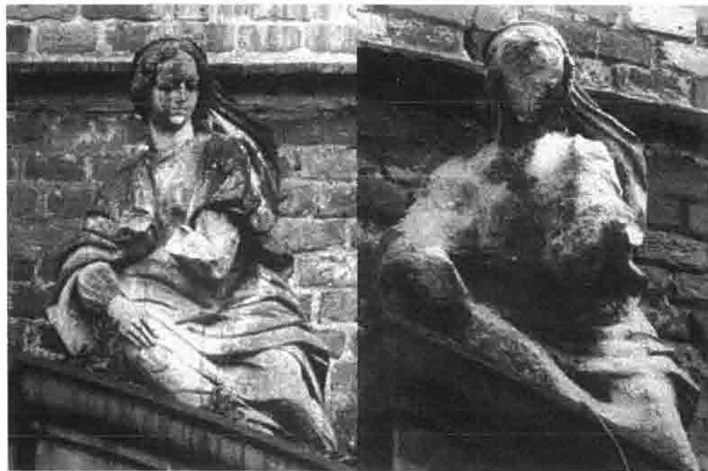
How acid rain affects stonework. The picture on the left was taken in 1908. The picture on the right was taken in 1968.
