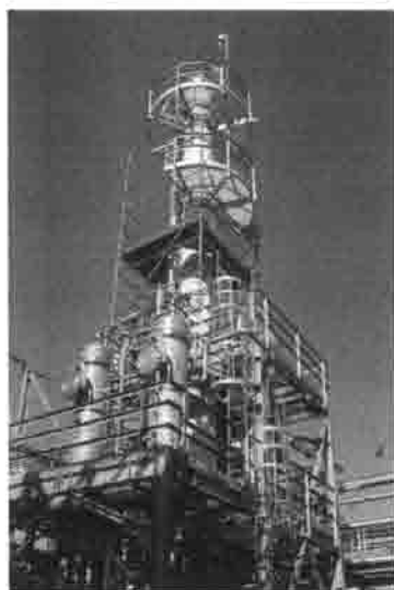
Spent Acid Regen Tail Gas 36 MMSCFD
