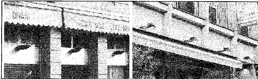
Fig.21 - Left: a shop window incorrectly lit up from the bottom to the top. Right: the lighting is corresponding to the R.L. 17/00 requirements. If the right shop window was truly conform, it would not need neither a project nor authorization by the competent authority.
