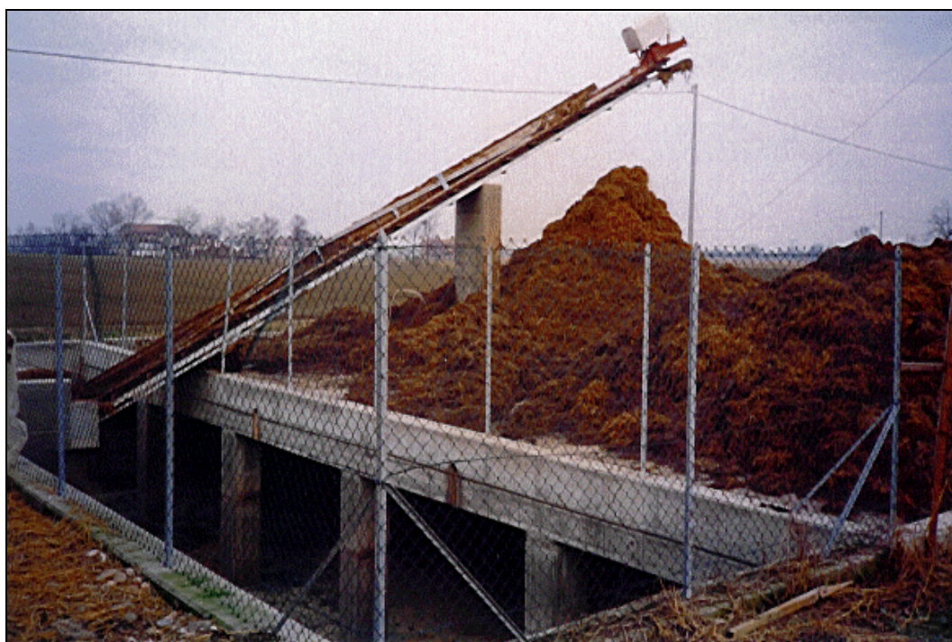
Figure 2.33: Storage of littered manure with separate containment of the liquid fraction (Italy)
