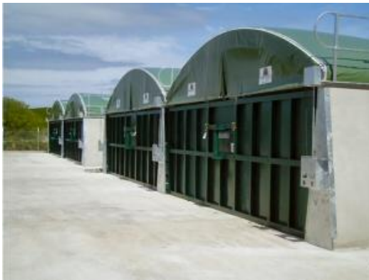
Photograph 4.11: A and B – Example of Sliding Roof Tunnel System
