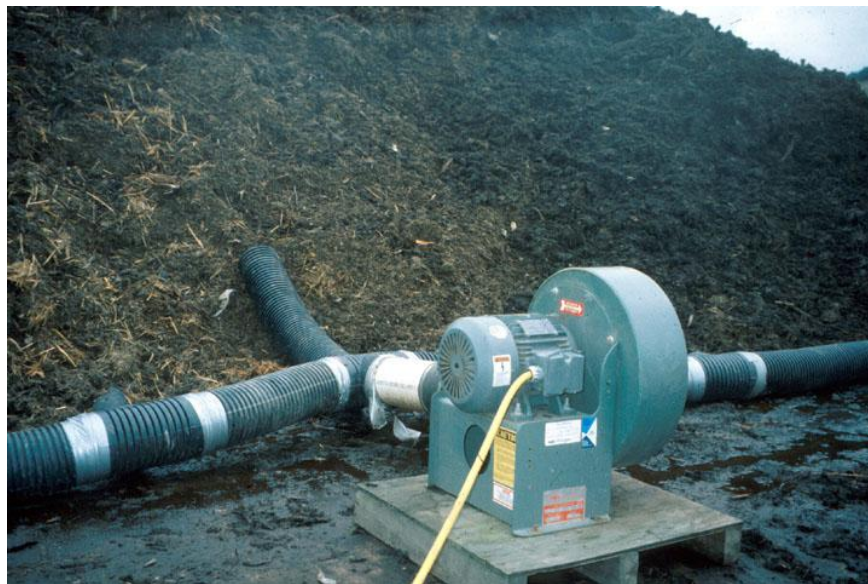
Photograph 4.9: Aeration Supply to an Aerated Static Pile
