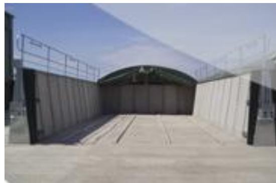
Photograph 4.11: A and B – Example of Sliding Roof Tunnel System
